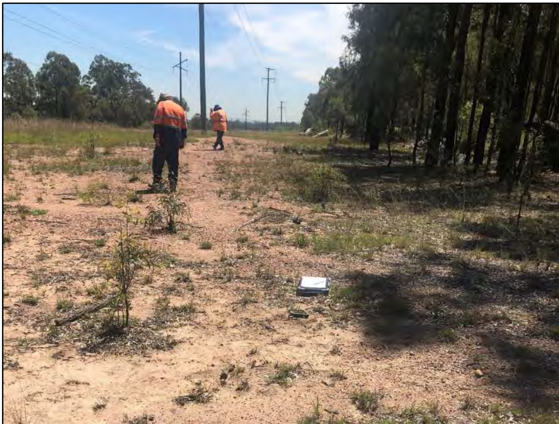
View north through HVO-1534 within power-line easement
